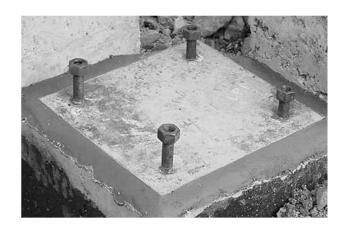
ASTM F1554 Anchor Bolts [Grade 36, Grade 55, Grade 105]
